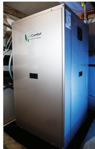
Right: The GeoComfort Variable Speed Water-to-Water unit, nestled under the lower level switch back staircase of the home.
