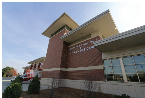
Clockwise from top Right: Four 20-ton WD systems heat and cool the building Outdoor portions of the fire and EMS station
