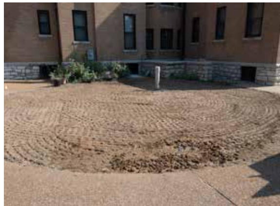
Left: Work continues on the loop installation.
