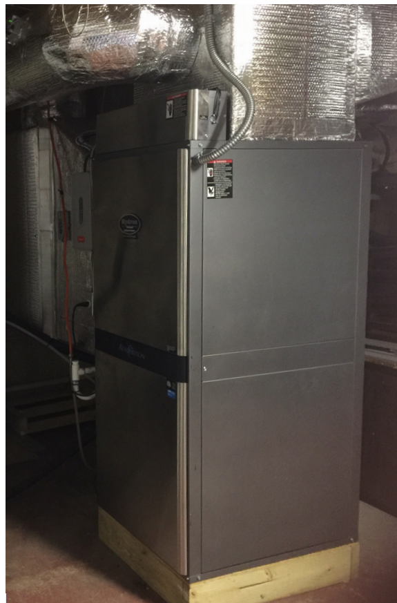
Left: The loops were installed in vertical wells
