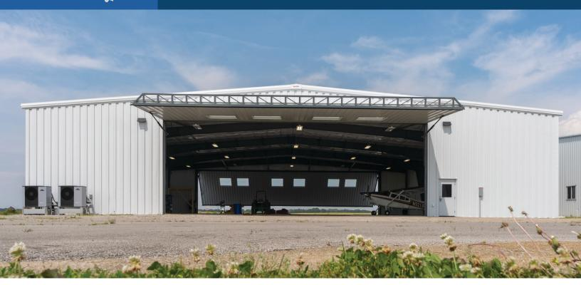
Greenville Airport is opening the doors to new possibilities with radiant heating powered by Enertech's Advantage air-to-water heat pump. The goal: to go all-electric while maintaining a comfortable working environment. Radiant in-floor heating does just that by keeping the floors warm and reducing the recovery time that comes with opening and closing a 70 ft. wide hanger door.
